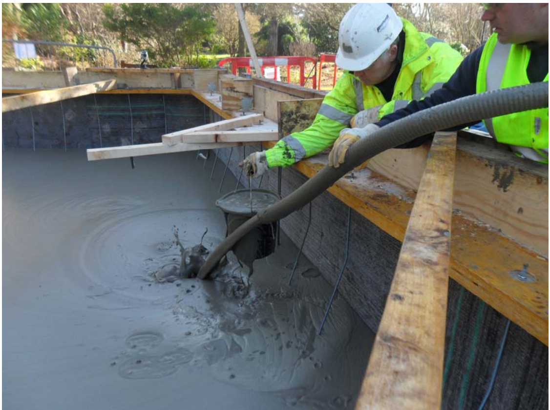
Figure 21: Pouring the aerated concrete slab.
