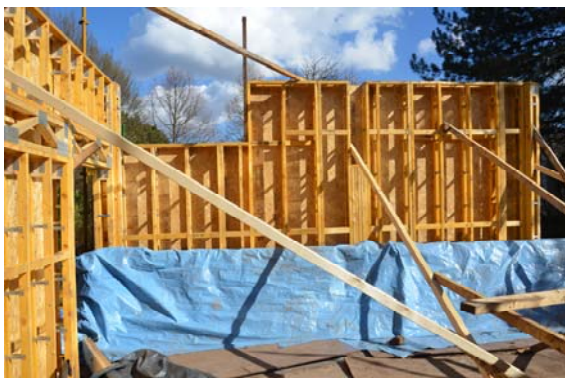
Figure 15: SpaceStud used in the wall construction
