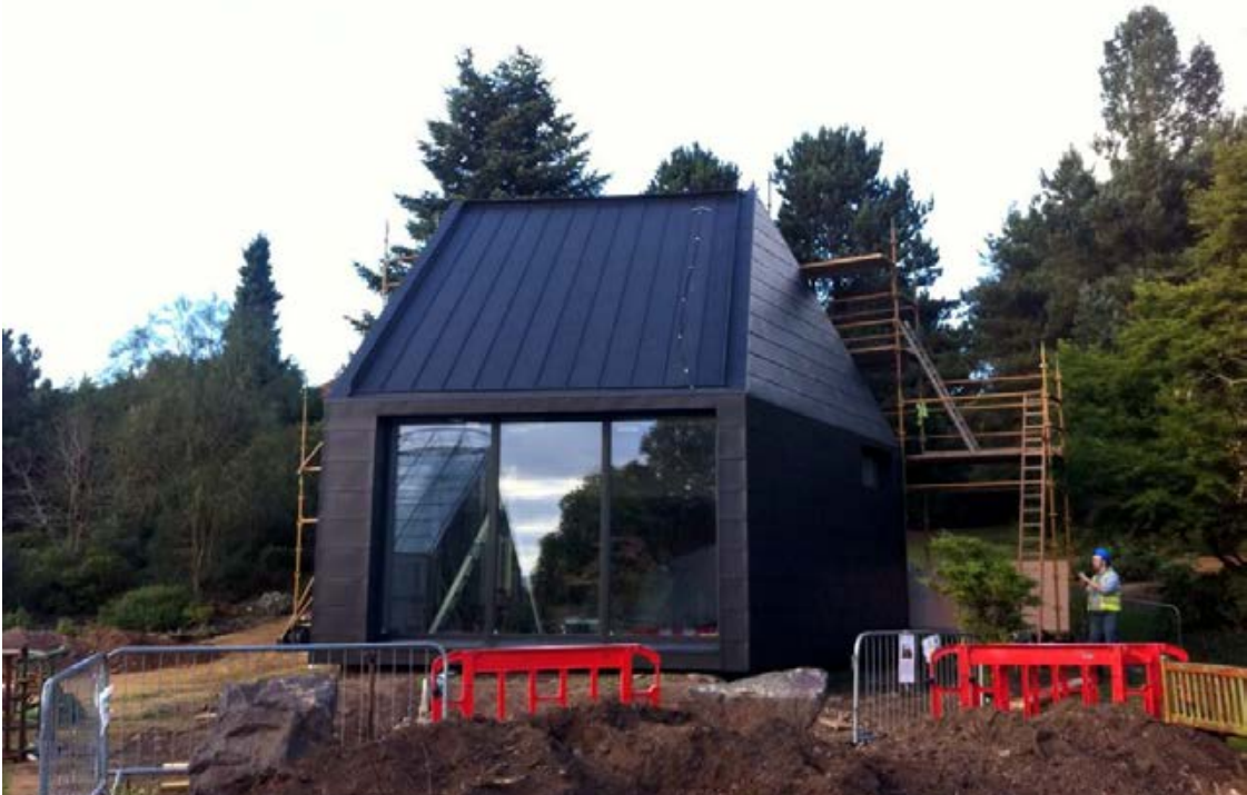
Figure 3: View from South East
