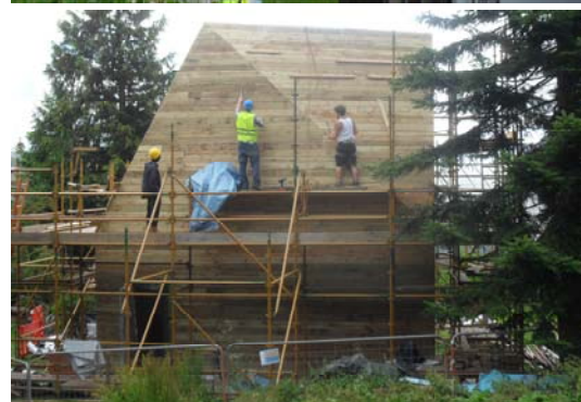
Figure 24: Construction of the roof onsite
