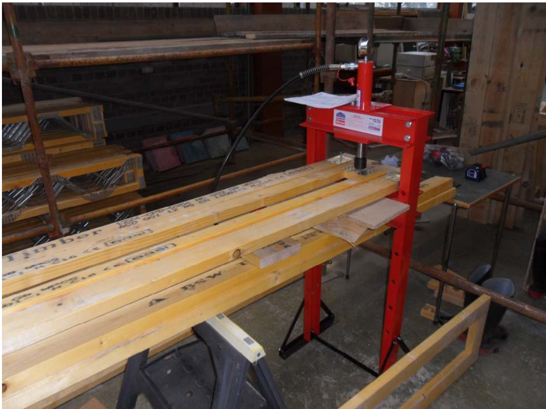
Figure 17: Manufacture of the wall cassettes in Fulton Structures Laboratory
