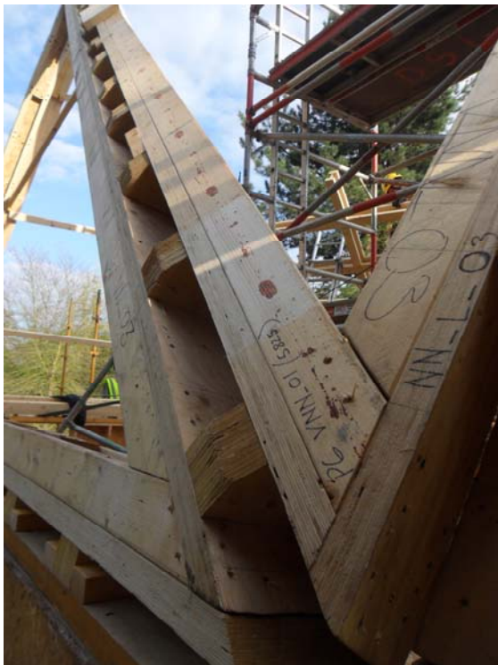
Figure 23: Roof plate Connections Installed
